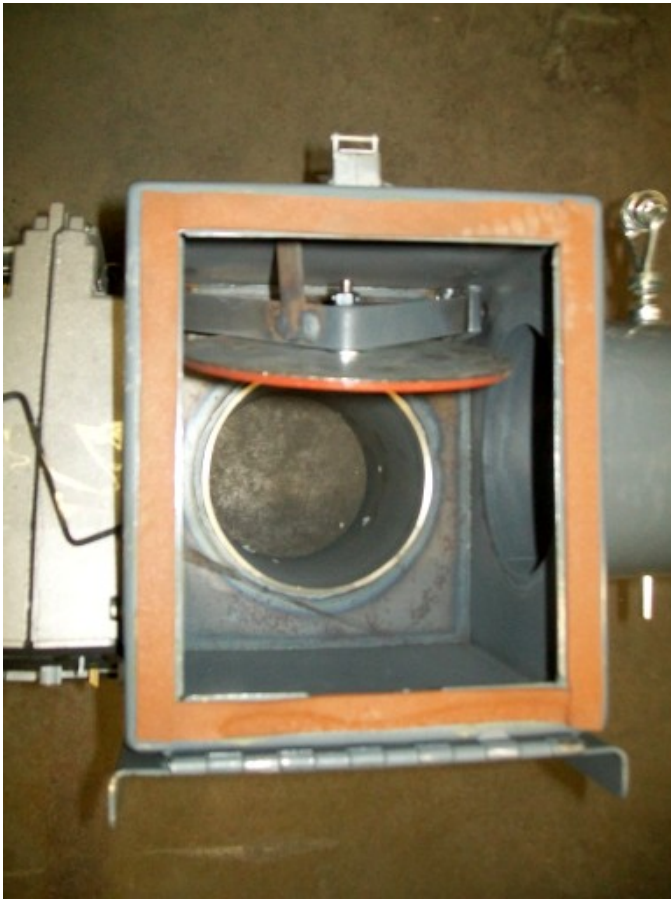
Air Valve Disk in Open Positioning
