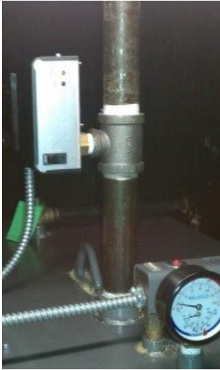
Photo: Low Water Cutoff Installation
