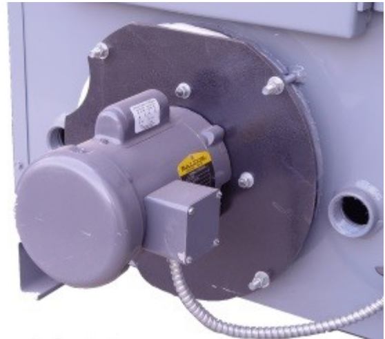
Direct-drive fan attached to boiler
